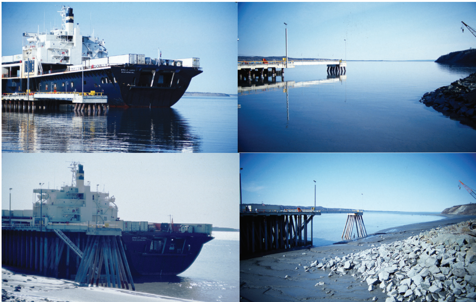
These two sets of photographs were taken from the same location 6 h apart at the port of Anchorage, Alaska, at approximately high tide and low tide. The tidal range this day was almost 11 m. For scale, note the cargo containers on the stern of the ship. They are the type hauled on 18-wheel trucks or flatbed railcars.
